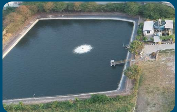
Fasilitas Clean Water Treatment
